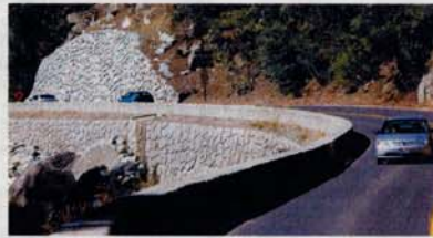
A newly built retaining wall is made of granite and materials that blend in with the surroundings.
